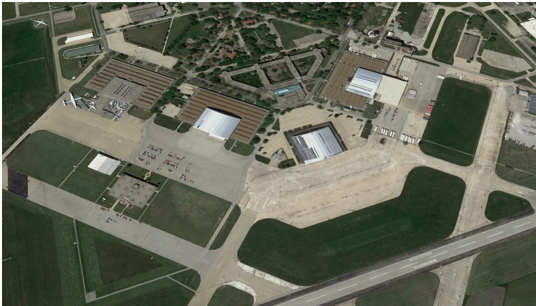
Aerial view of the four large hangars, the ramp areas, and one of the runways.
