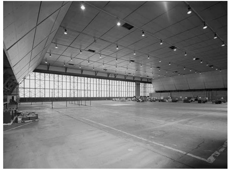
Aircraft hangar interior showing the 44' tall ceiling.
