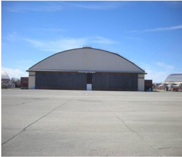
Aircraft hangar exterior with large ramp.
